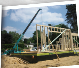
Timber Frame Work
